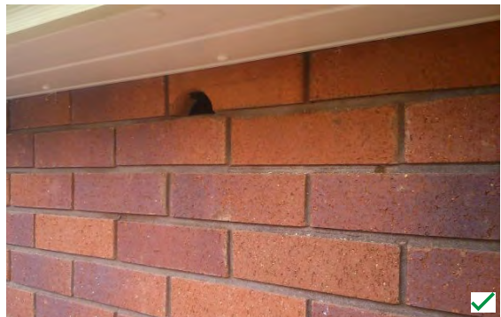
Figure 4.139: Example of an integrated bird box
