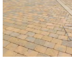
Mixed buff tegula paving, stretcher bond
