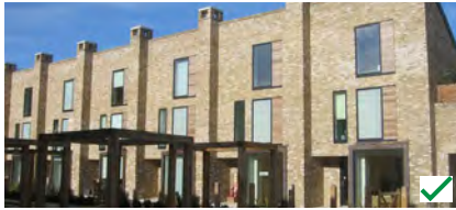
Principal material take through the entire building and through a group of houses
