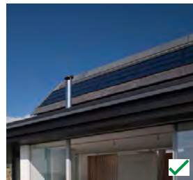
Figure 5.82: Solar/PV panels integrated into building design
