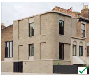
Figure 5.24 - Good example of a dual aspect house which successfully addresses both streets
