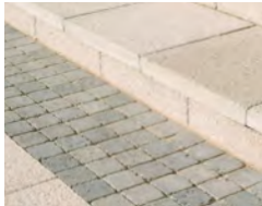
Mixed grey tegula setts, stretcher bond
