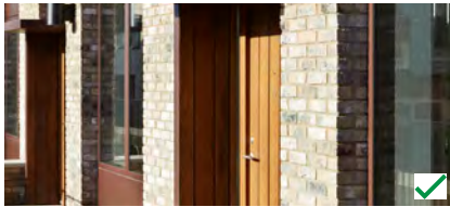
Full brick window reveals give a sense of depth
