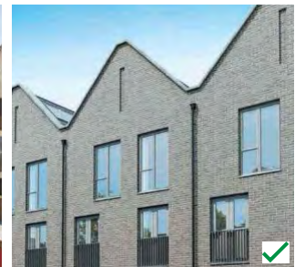
Figure 5.68: Example of carefully detailed building that create a clean and uncluttered elevation
