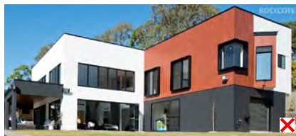
Lack of consistency in use of material and detailing within the same building
