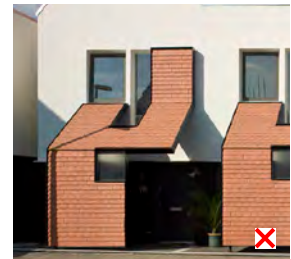
Figure 5.53: Porch materials do not match the materials used on the building
