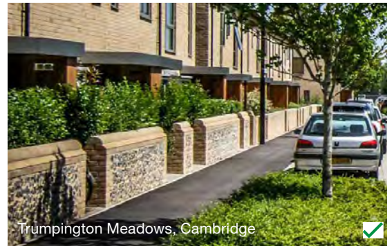
Figure 5.42: The consistent use of a low wall and hedge creates a clear, orderly character of street front
