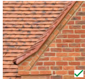
Figure 5.60: Brick detail is simple and the same colour as the facade
