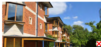
Contrasting, thick window frame sections
