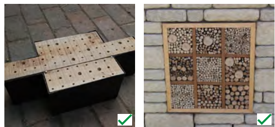
Figure 4.141: Example of integrated insect boxes
