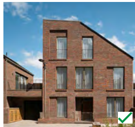
Figure 5.52: Porch designed as integral to the elevation which provides sufficient shelter
