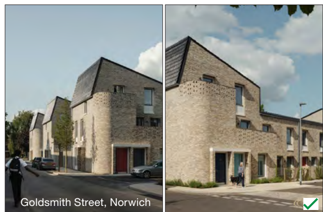
Figure 5.27 - Example of corner building (split into flats) that integrates/ complements and continues both frontages in a successful way, even though frontages have different requirements in terms of scale, height, boundary typologies etc
