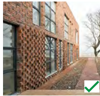
Brick detailing adds texture and interest
