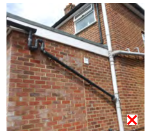
Figure 5.63: Rainwater pipes dominating the elevation
