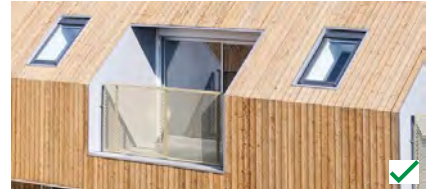
Using the same material for roofs and walls to express the geometry of the building
