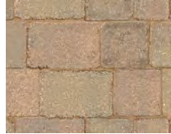
Buff tegula paving, stretcher bond
