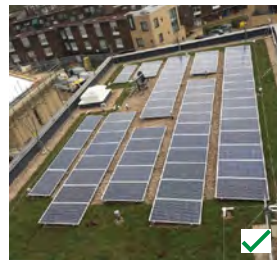
Figure 5.54: Flat roofs should have a sufficiently high parapet to hide the photovoltaic panels
