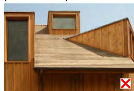
Figure 5.56: Dormer windows and inconsistent roof pitches
