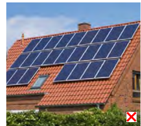
Figure 5.55: Photovoltaic panels must be designed into the elevation
