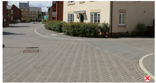
Figure 4.135: Junctions and crossing points without tree planting can feel vehicle focused and hostile
