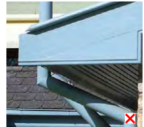
Figure 5.61: Boxed eaves are not permitted
