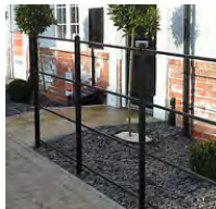
Metal railings (horizontal)
