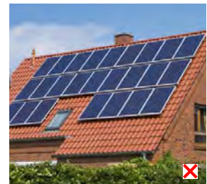
Figure 5.83: Solar panels detracting from building design
