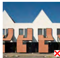
Pastiche elements that contradict the building geometry
