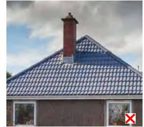
Figure 5.59: Chimneys should be positioned symmetrically to ridge
