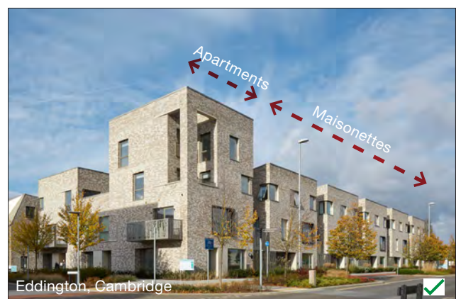
Figure 5.30 - Example of a podium building that integrates both flats and maisonettes, with a consistent and complementary architectural approach. Each side has slightly different requirements in terms of boundary typologies at the ground floor, street activation and privacy, but the building creates a consistent rhythm and uses the same materials. The corner is expressed through a slightly increased height
