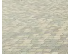
Mixed grey tegula paving, stretcher bond
