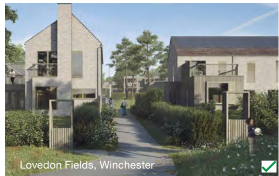
Figure 5.46: The use of a low hedge and a timber gate for rear boundaries of dwellings which face less formal public open space (3c)
