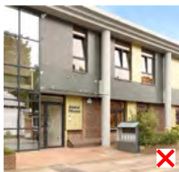
Unnecessary use of too many materials
