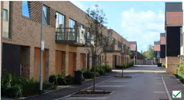
Figure 4.132: Tertiary street tree planting located closer to buildings but fastigiate in form so as not to encroach within 2m of building facades
